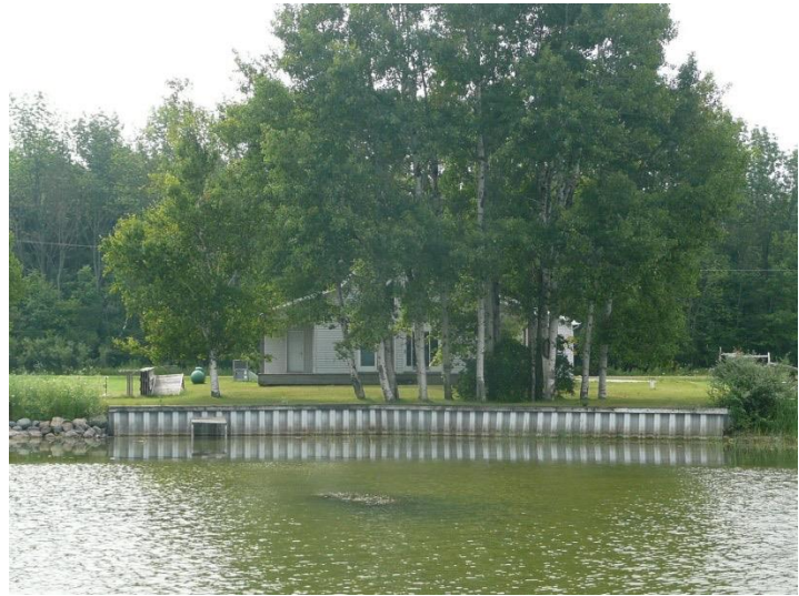
Example of retaining wall
