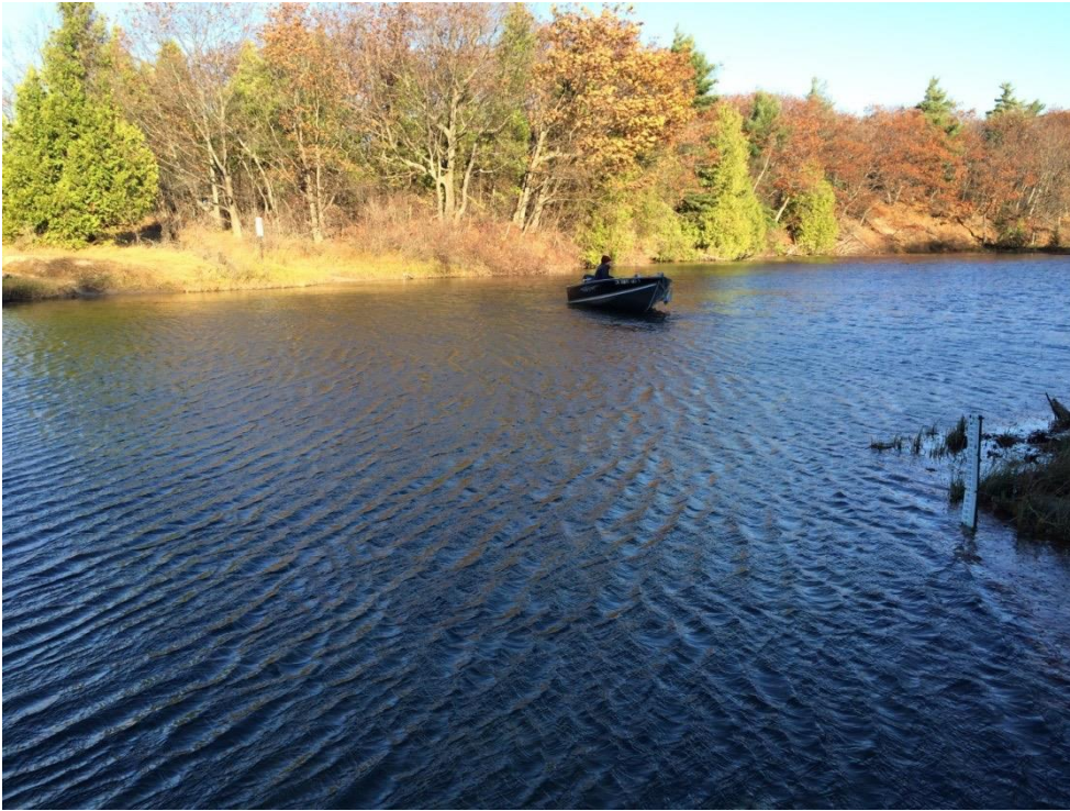
Lower Herring Lake Outlet at Lake Michigan, looking north from outlet flow control structure.
