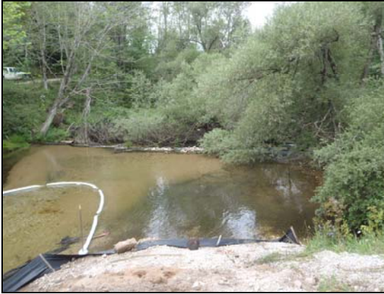
Before-looking downstream from Bridge construction site
