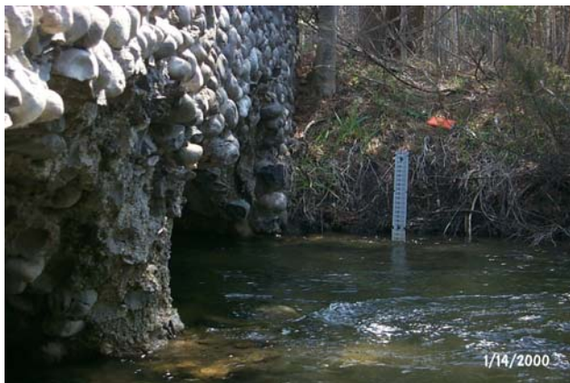
Platte River, Stone Bridge
